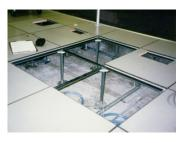
Raised floors are traditionally 12-15" off the physical floor. They are constructed of interlocking metal chassis and struts with removable tiles and grommets. The grommets (pictured to the right) provide
